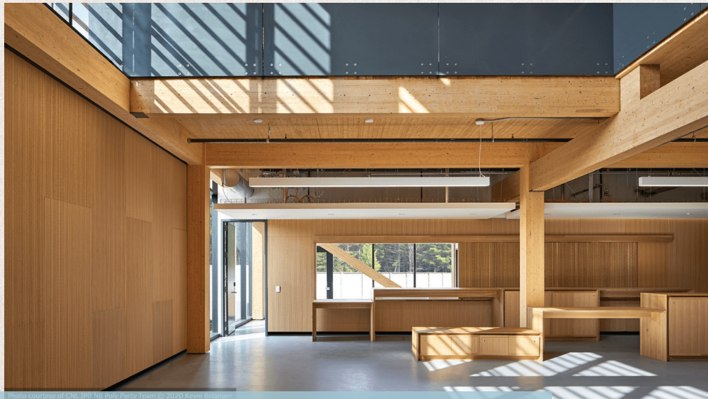
Photo courtesy of CNL IRO NS Policy Party team © 2020 Kevin Bellinger Mass timber project at Chalk River Laboratories, Ontario, Canada. Credit: Nordic Structures
